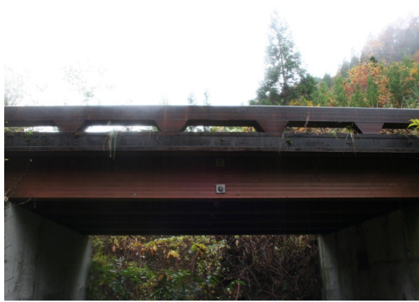
坊川林道二号橋
